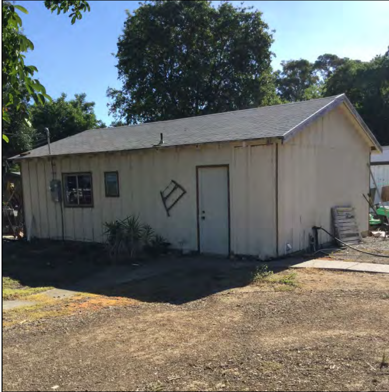
Figure 12. Garage (FAC-004) overview (view northeast) June 15, 2017.
