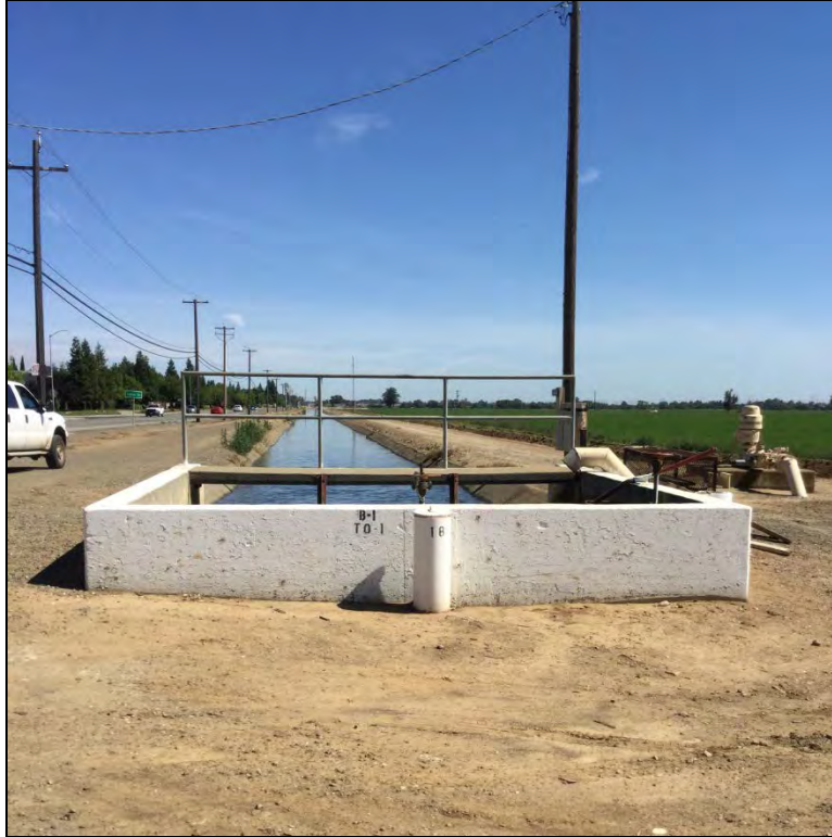
Figure 11. Byrnes Canal (FAC-001) overview from southwest corner (view north) June 15, 2017.
