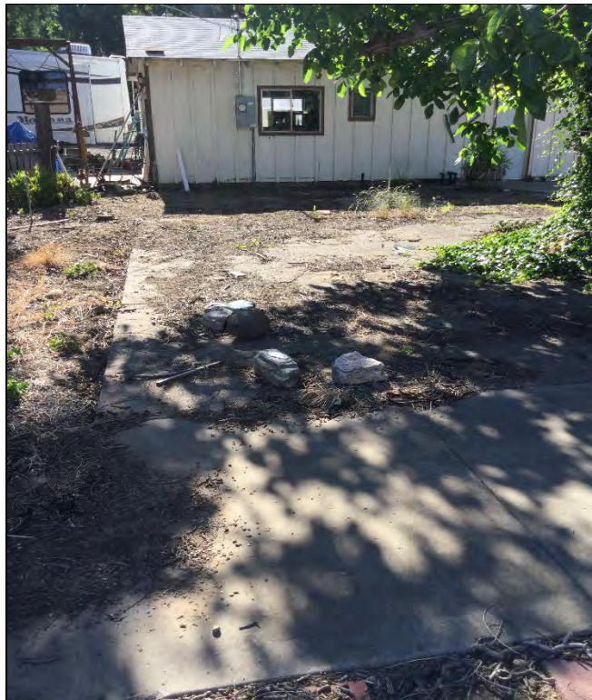
Figure 13. Concrete foundation next to garage (view east). June 15, 2017.
