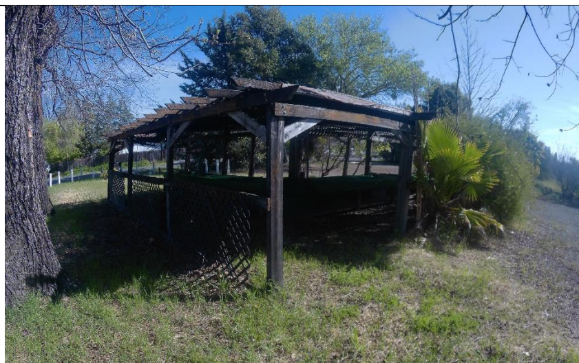
Figure 16. Structure 11 (view to north_IMG 72)
