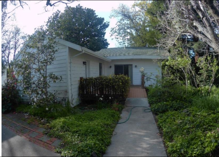
Figure 5. Main elevation of Residence 2 (View to South_IMG 2)
