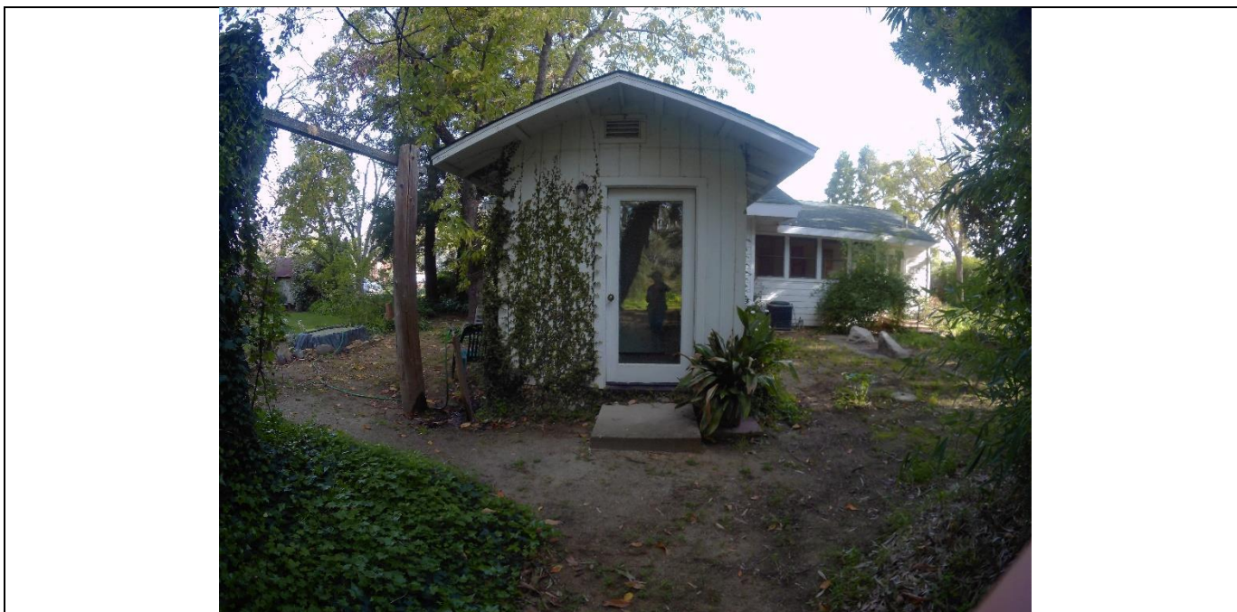
Figure 7. Structure 2 (view to north_IMG 13)
