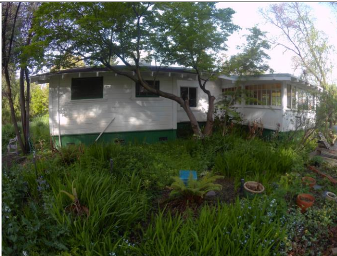
Photograph 1. Rear Elevation of Residence 2 - View to West (Image # IMG_21)
