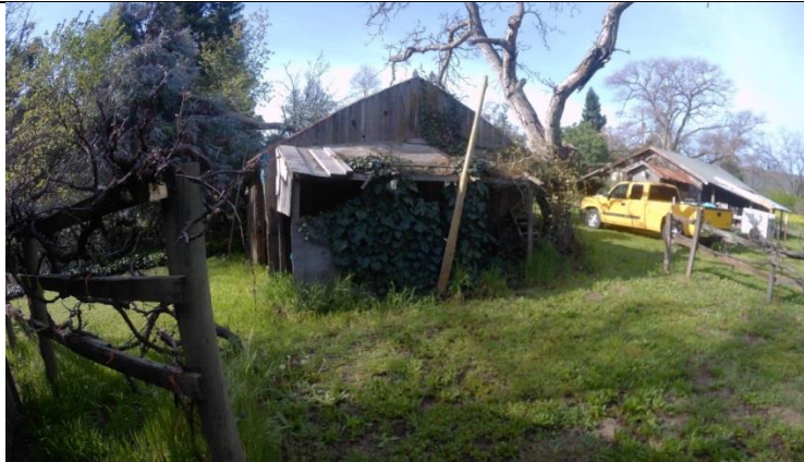
Photograph 5. Structure 8 - View to Southwest (Image # IMG_57)
