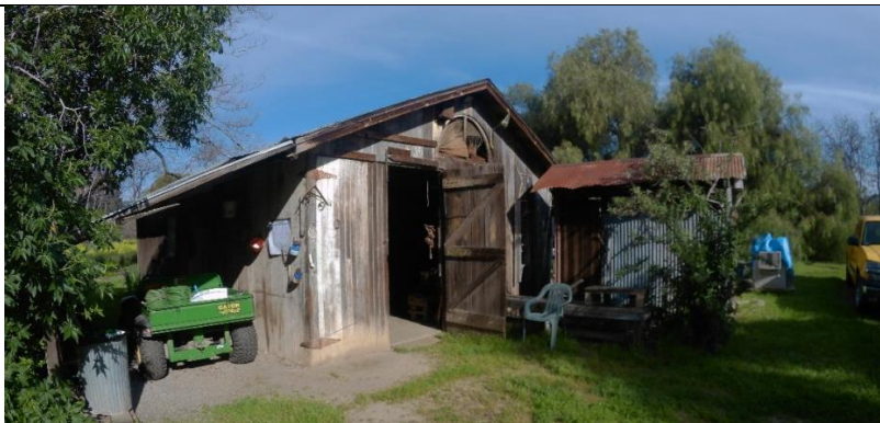
Photograph 4. Structure 5 - View to Northwest (Image # IMG_48)
