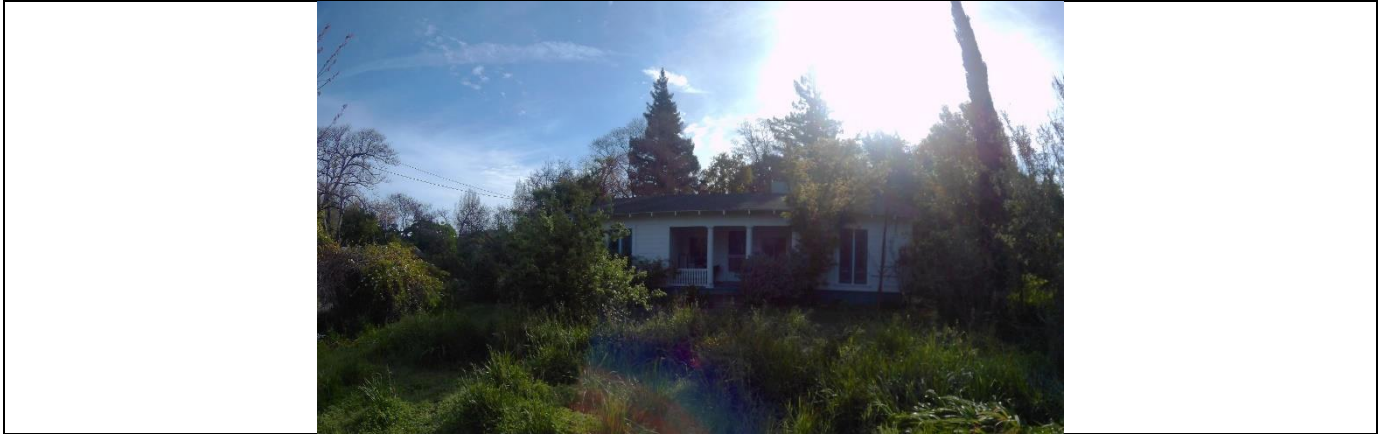
Figure 4. Main elevation of Residence 1 (View to east_IMG 23)
