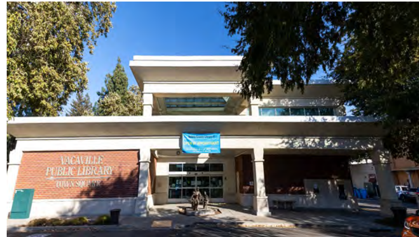
Town Square Library in Downtown Vacaville (Source: ESA)
