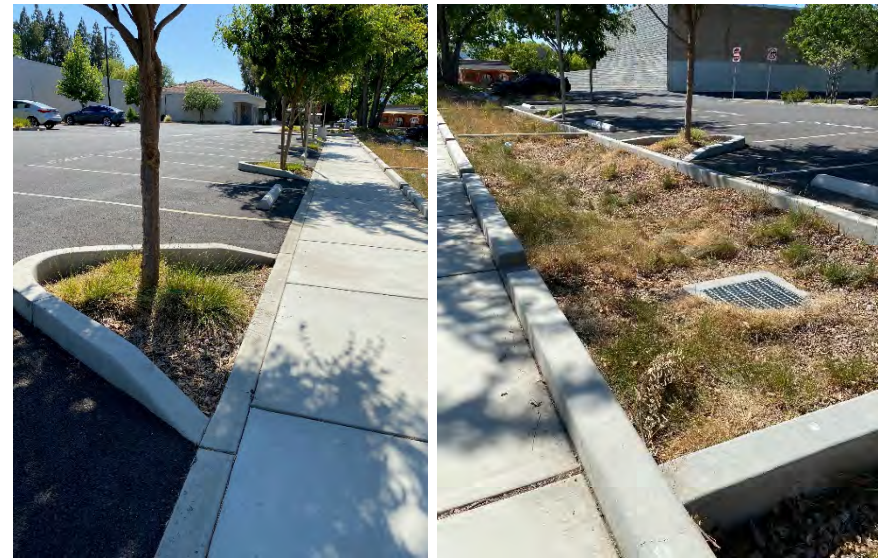
Bioretention in a parking lot
