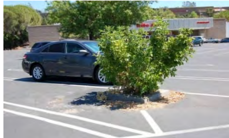
Parking lot island of inadequate size and design (Source: Jacobs)
