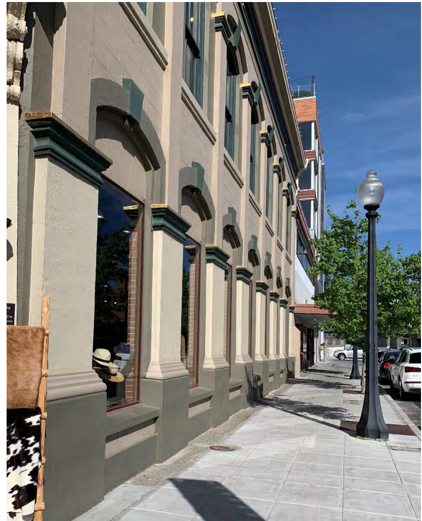
Example of a continuous street wall in Downtown Napa (Source: ESA)
