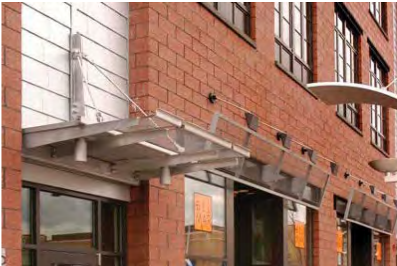
Example of appropriate building materials—brick and steel (Source: Jacobs)
