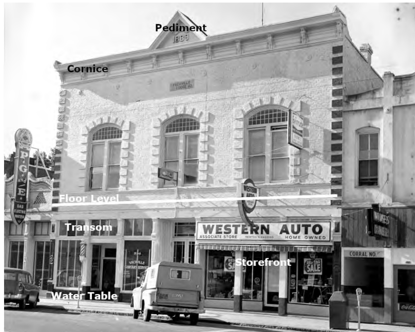
Parts of a building façade (Source: Vacaville Heritage Council)
