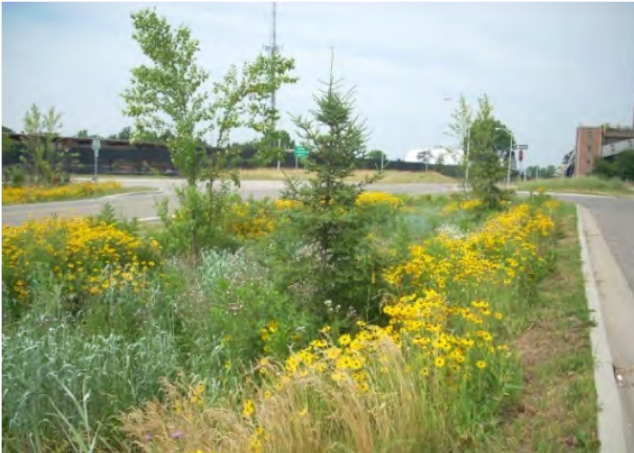
Figure 54 Flow-through stormwater planter
