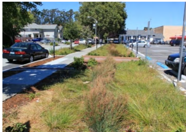
Figure 56 Street-side stormwater bio-retention area
