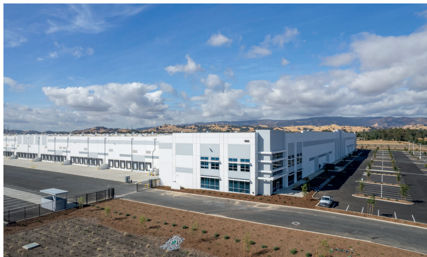
Midway Commerce Center Building A 198,490 SF.
