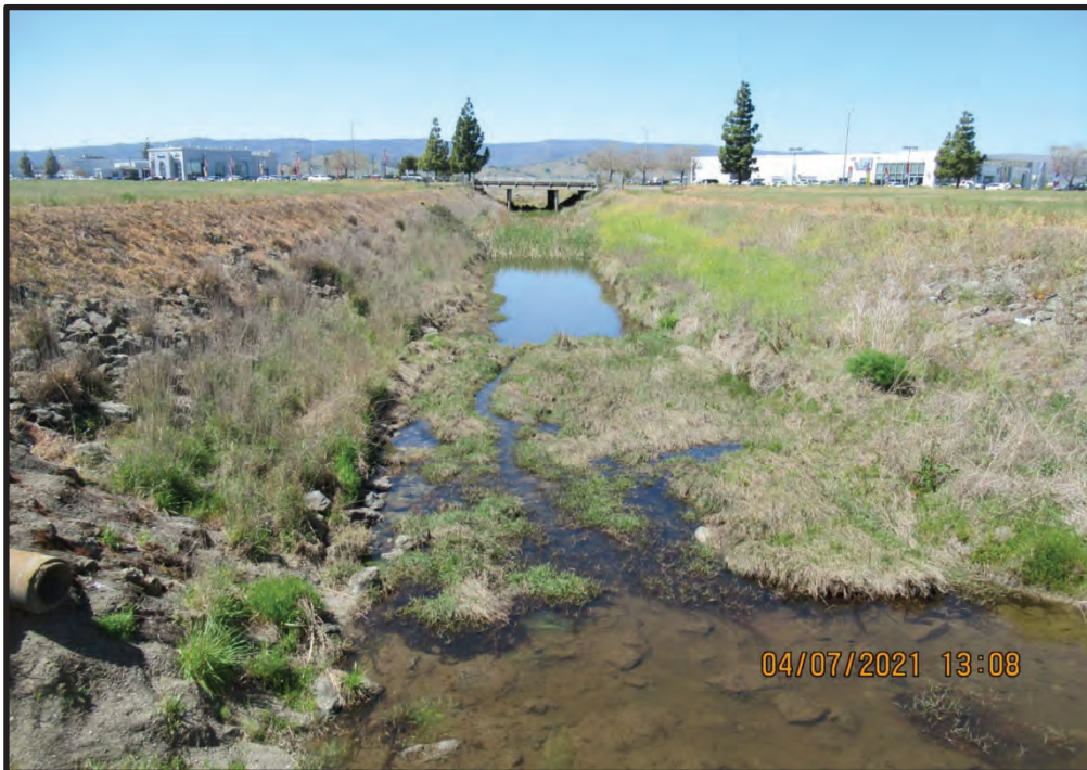
Horse Creek, which is adjacent to the north edge of the site, looking west; 04/07/21. Treated storm water from the north part of the Greentree Project will discharge to Horse Creek via an existing outfall.
