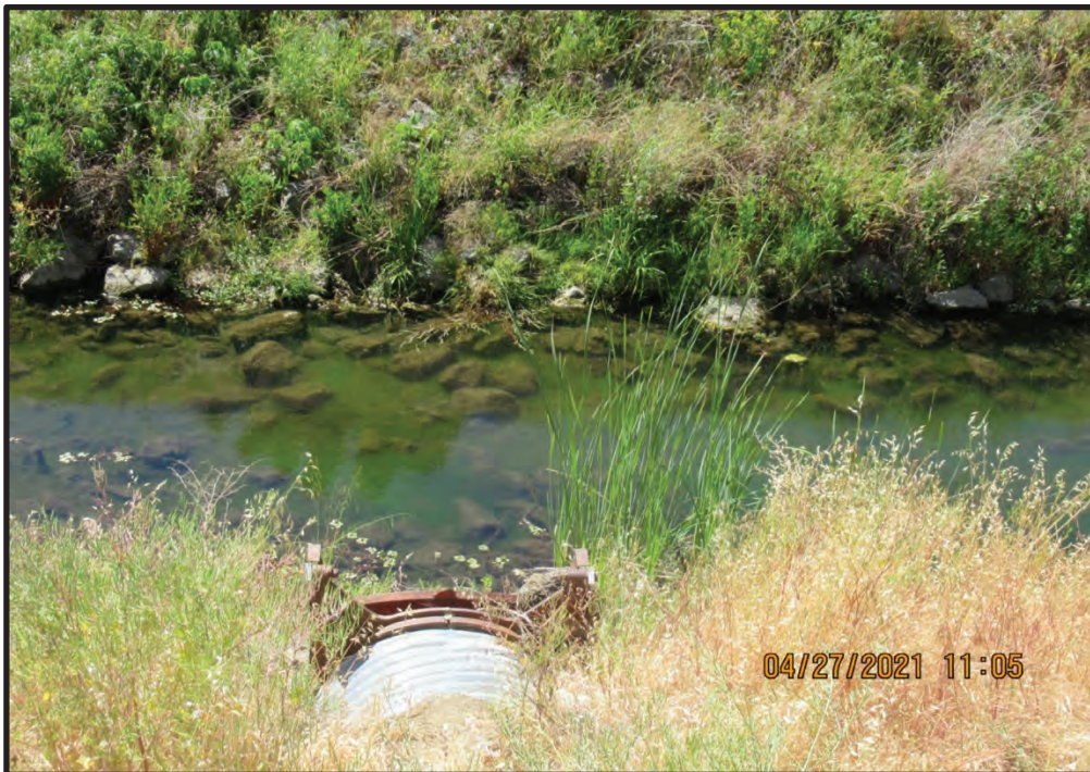
Storm drain outfall in Ulatis Creek adjacent to the southwest corner of the site, looking southeast; 04/27/21. Treated storm water from the southwest part of the Greentree Project will be discharged through this outfall.
