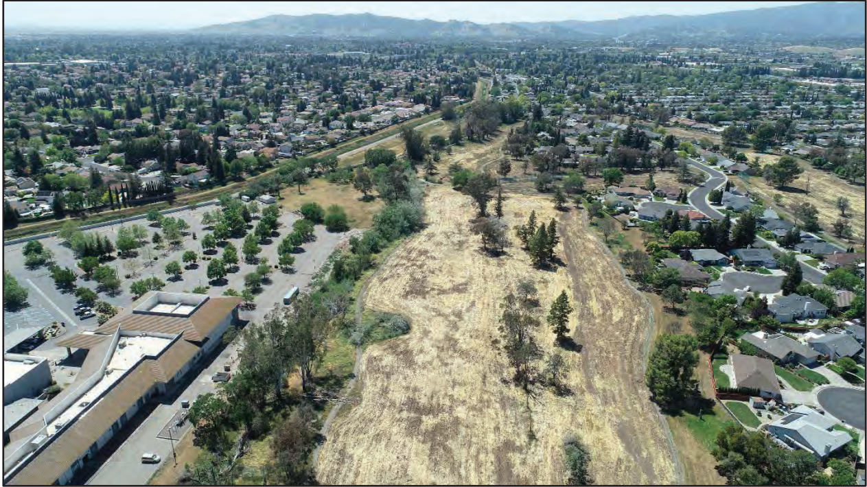
Looking southwest over southern portion of the study area. Photo Date 4-16-21
