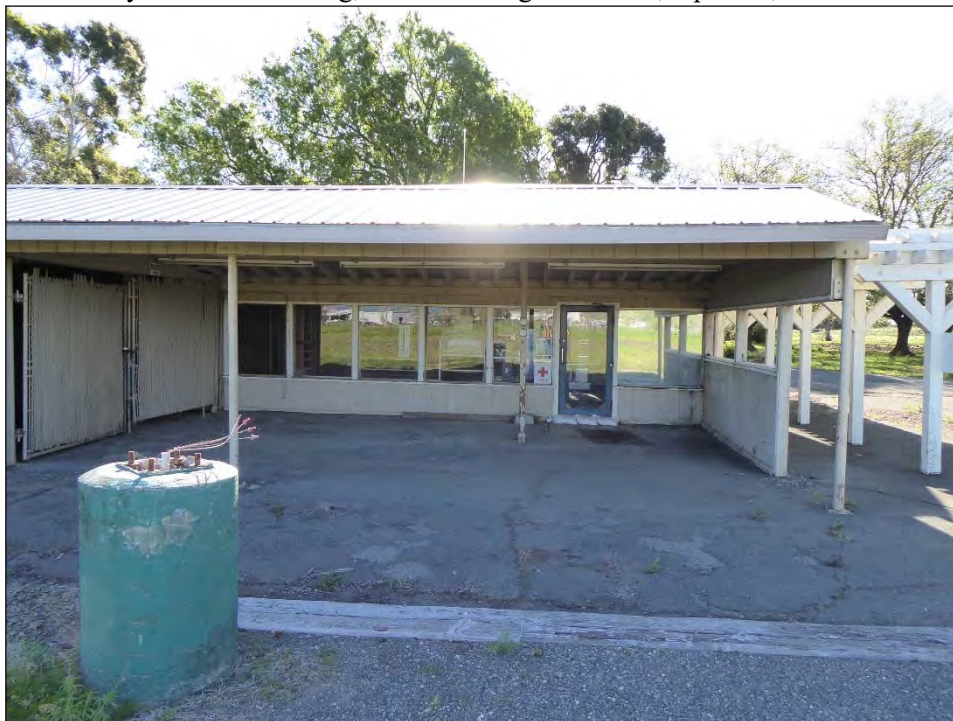
Photograph 11: Golf cart staging area, showing the fenestration of the west side of the clubhouse, camera facing east, April 12, 2019.
