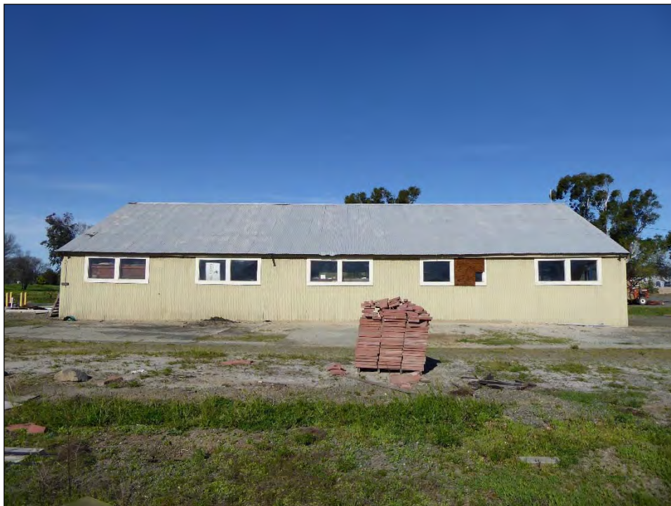
Photograph 17: Warehouse rear (east side), camera facing west, April 12, 2019.
