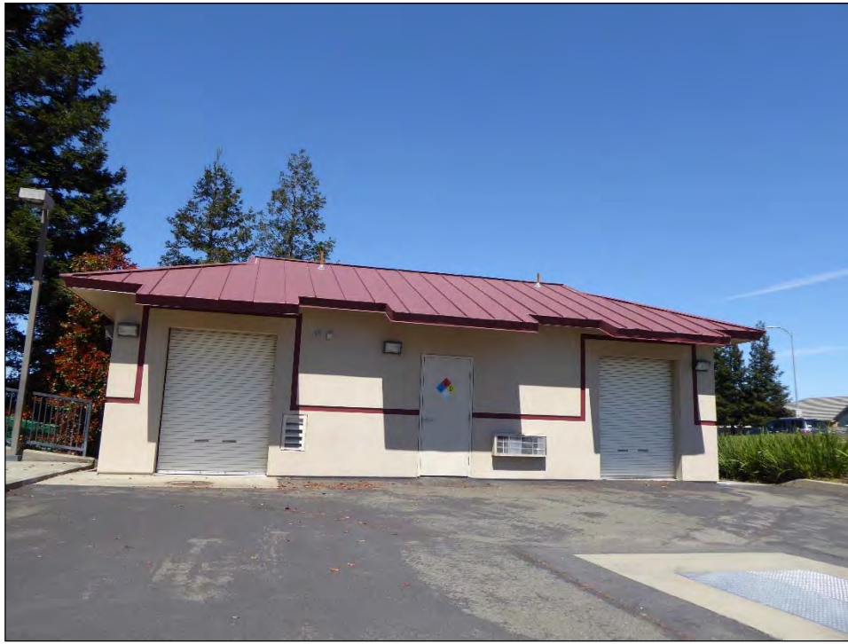
Photograph 34: Sewer lift station, camera facing north, April 12, 2019.
