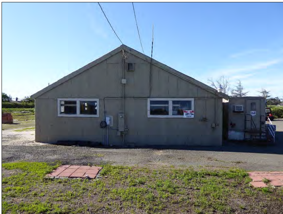
Photograph 15: Warehouse, north gable end, facing south, April 12, 2019.
