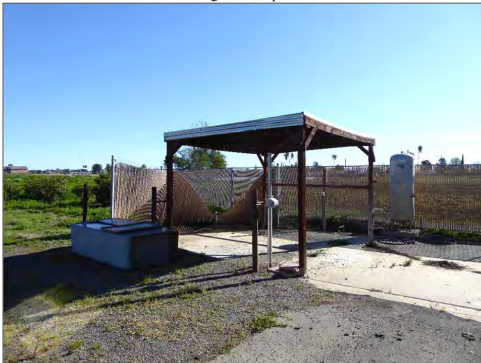
Photograph 13: Wood-frame shelter located northeast of the clubhouse and golf cart storage structure, camera facing northeast, April 12, 2019.
