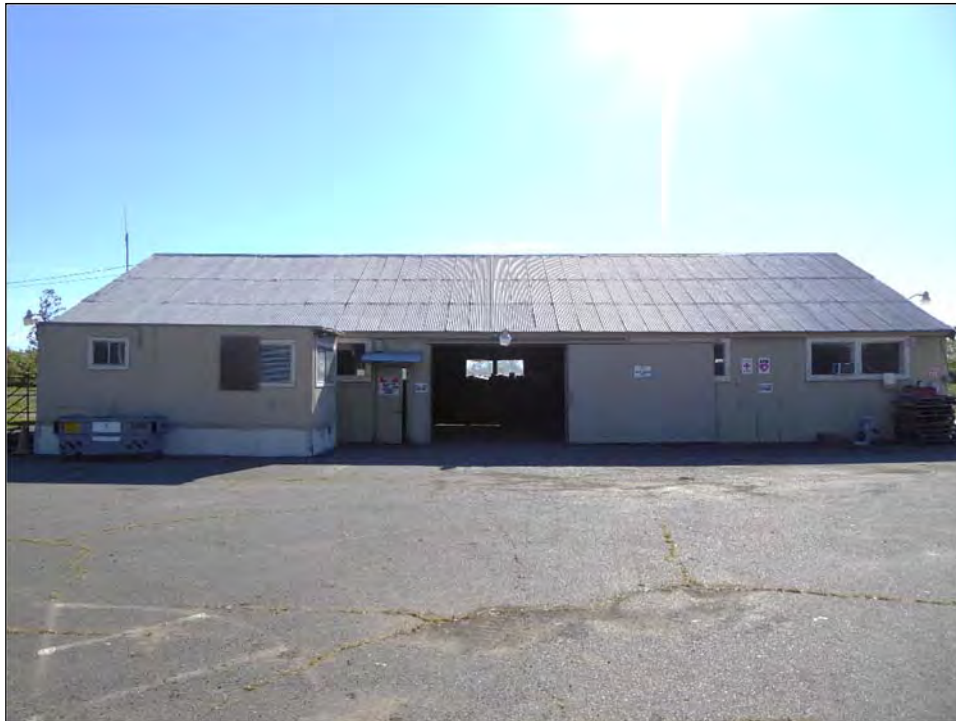
Photograph 14: Warehouse primary façade, camera facing east, April 12, 2019.
