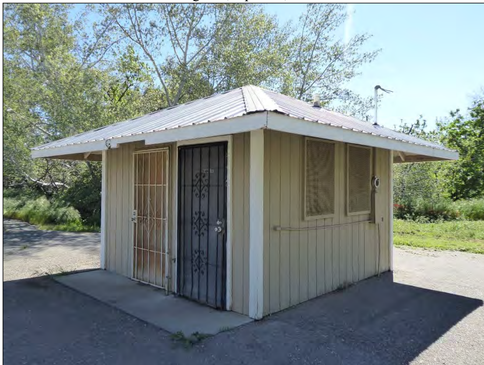
Photograph 33: View of a restroom near Hole 15, camera facing northeast, April 12, 2019.
