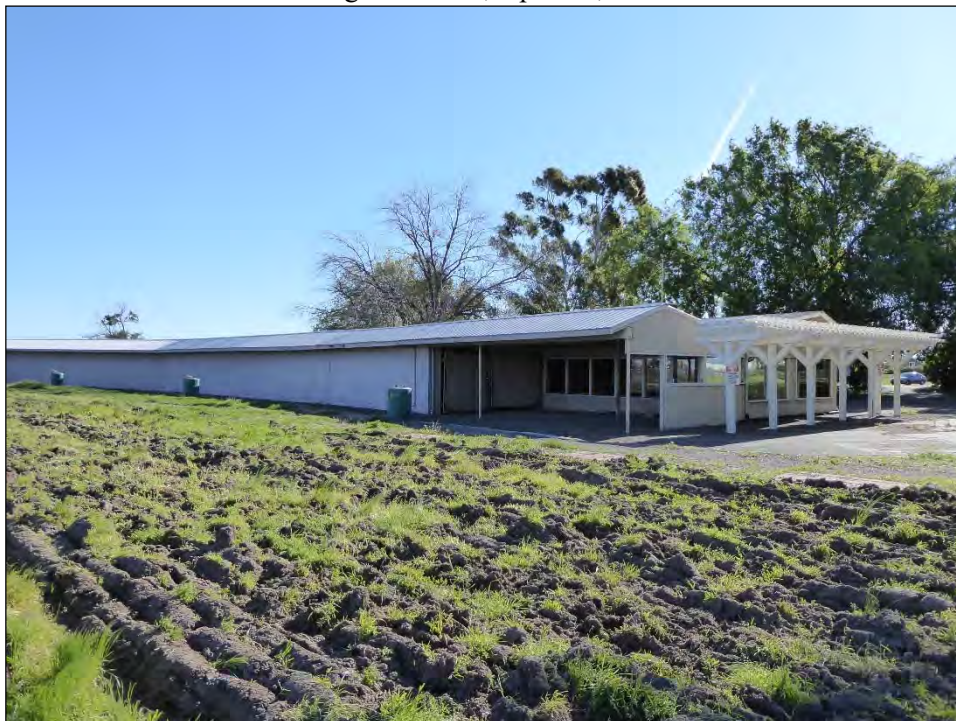
Photograph 9: View of the west side of the golf cart storage structure, enclosed by plywood, camera facing northeast, April 12, 2019.
