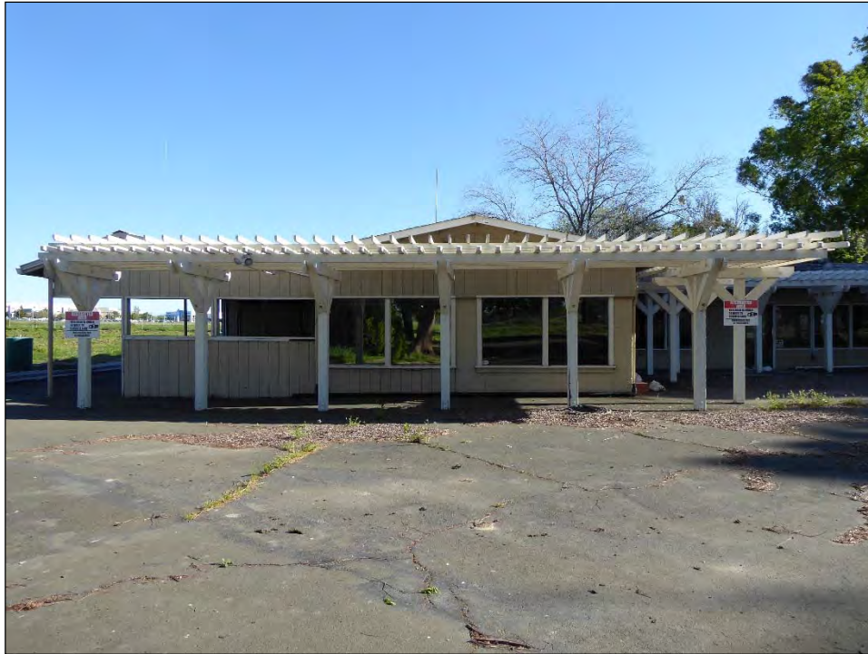
Photograph 4: Clubhouse south gable end, camera facing north, April 12, 2019.
