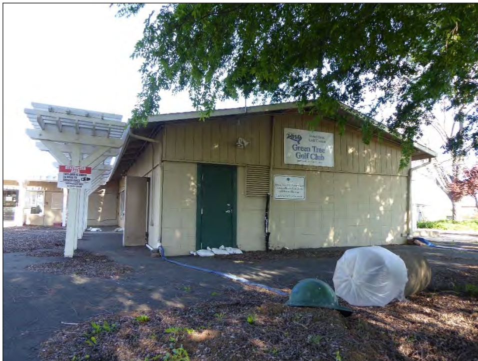
Photograph 5: Clubhouse east gable end, camera facing west, April 12, 2019.
