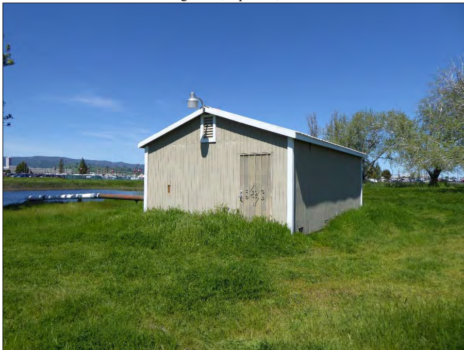
Photograph 37: Pumphouse located on the 9-hole course reservoir, camera facing northwest, April 12, 2019.
