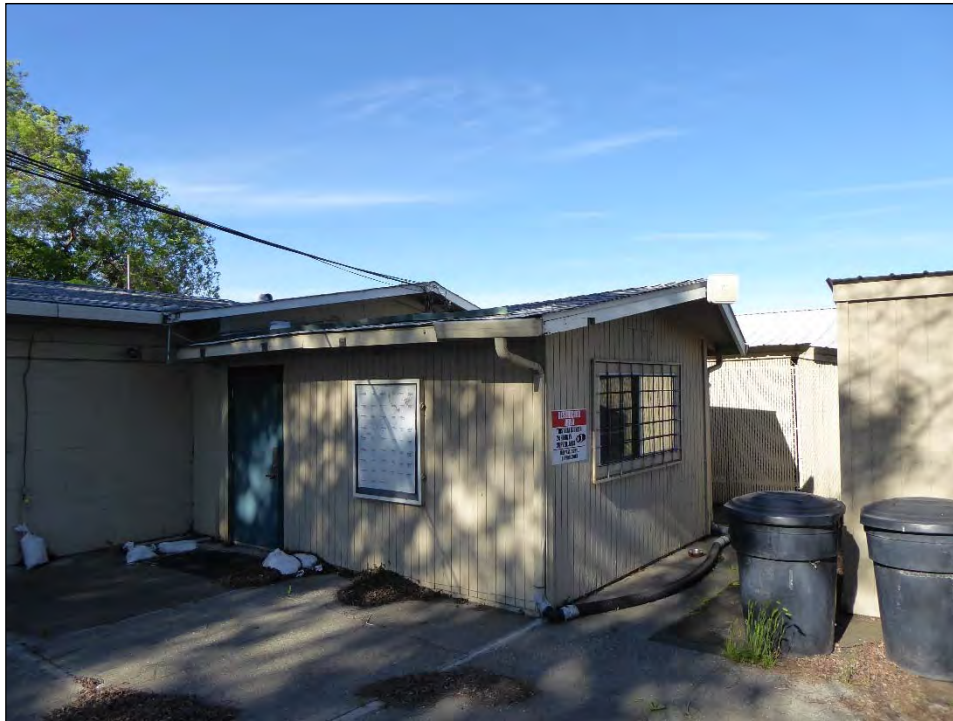
Photograph 6: North gable end of the clubhouse, obscured by modern addition, camera facing southwest, April 12, 2019.
