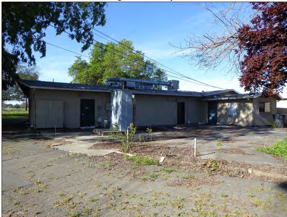
Photograph 7: Rear, north side of the clubhouse, showing the location of the modern addition, camera facing southwest, April 12, 2019.
