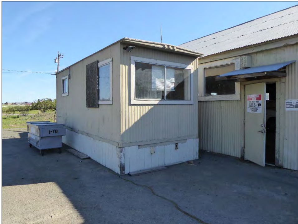
Photograph 18: Modular office, camera facing northeast, April 12, 2019.
