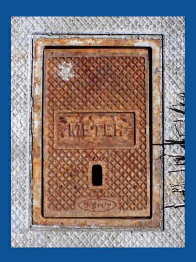
2. Use the hole in the water box lid to open the water meter box.
