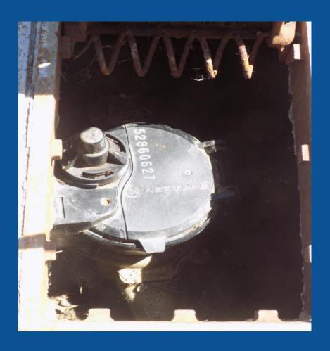
3. Lift the lid of the water meter. This will activate the light sensor on the meter and a set of numbers will appear on the LCD display. The first four numbers, all the way to the left, are your usage. The numbers are shown in units, or cubic feet. Each unit is 100 cubic feet, which is equal to 748 gallons.
