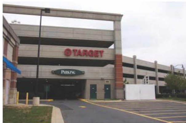
Washingtonian Center, a retail and entertainment center in Gaithersburg, Maryland, includes a large structured parking facility to accommodate the necessary parking. This view is of the back of the structure; the front of the structure incorporates retail uses on the first floors.
