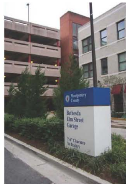
This parking structure in Bethesda, Maryland, is embedded in the block, obscured from street activity by more active uses.
