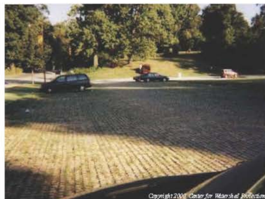
The use of alternative pavers in overflow areas reduces impervious surface coverage and helps facilitate groundwater recharge. Credit: Center for Watershed Protection
