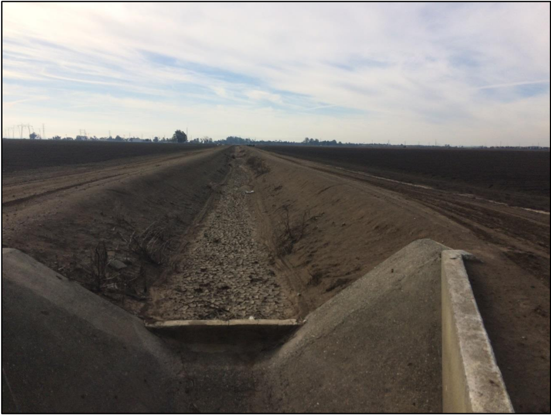
Photo Point 1: Facing South
