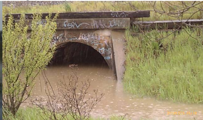
Existing culvert under Union Pacific Railroad R/W
