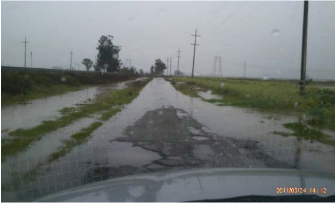
North of RR culvert looking southwest
